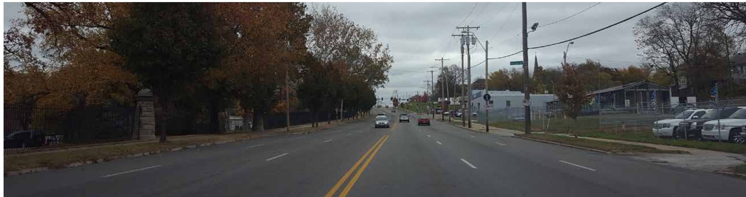
Figure 10. Truman Road's wide curb-to-curb widths and lack of pedestrian-oriented streetscape elements reduce pedestrian comfort along the corridor.
