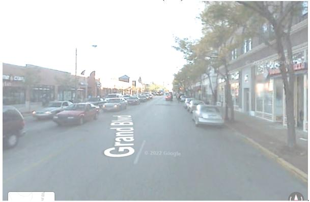
Four lanes plus parking, narrow sidewalk with narrow buffer
