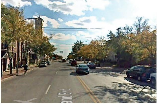
Four lanes plus parking, narrow sidewalk with narrow buffer
