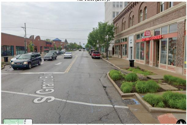
Two lanes plus center turn lane and parking, wider sidewalk and wider sidewalk buffer, landscaping. Traffic is calmed and much slower (25 mph speed limit) so that separate bicycle facilities are not necessary in this section now
